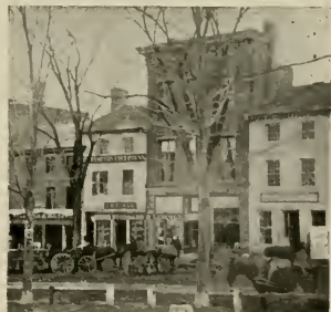
SHOP ROW, YEARS AGO
